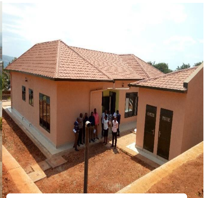
Rwinkwavu IOSC Shelter/safe house
