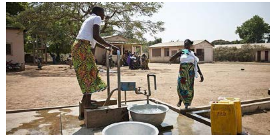
Drinking Water Supply in small town in Benin. (Photo: Swiss Water Partnership)
