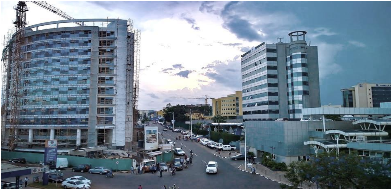
Housing in Kigali city
