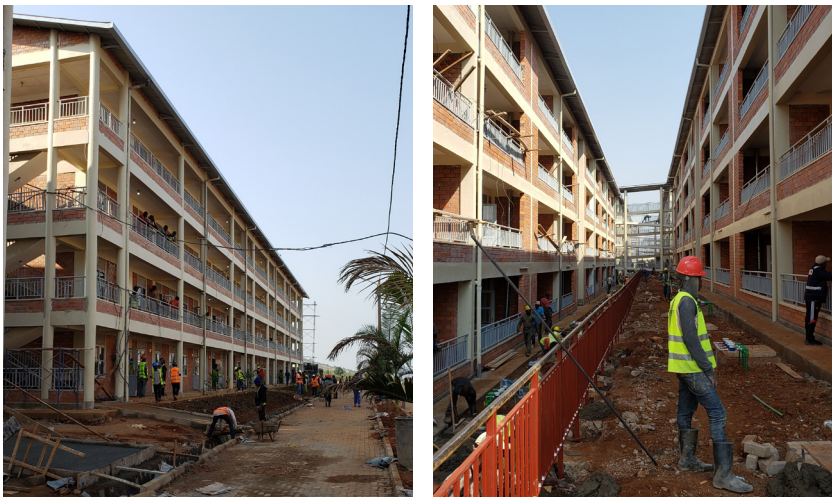
Model social housing complex in Karama, Kigali, Rwanda © Dheeraj Arrabothu
