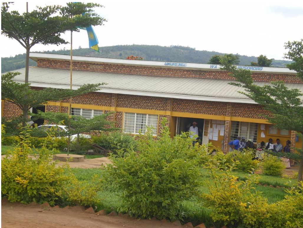
Picture 1.2: Building with no rainwater collection system
