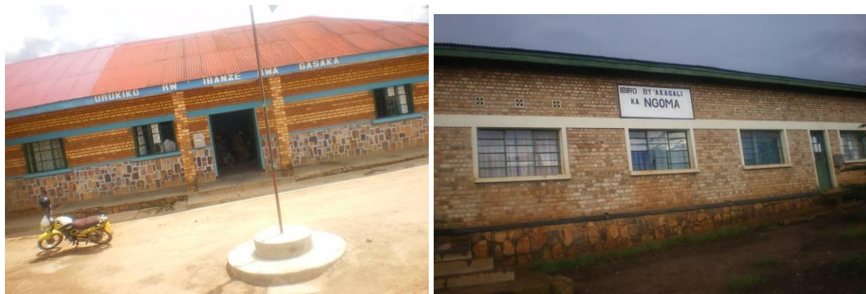
Picture 4.6: Simple isolated buildings - Gasaka and Ngoma offices in Huye sector
