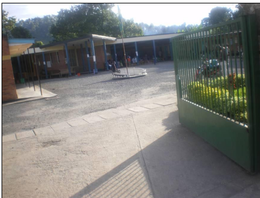
Picture 4.3: Muhoza Health Center – Northern Province
