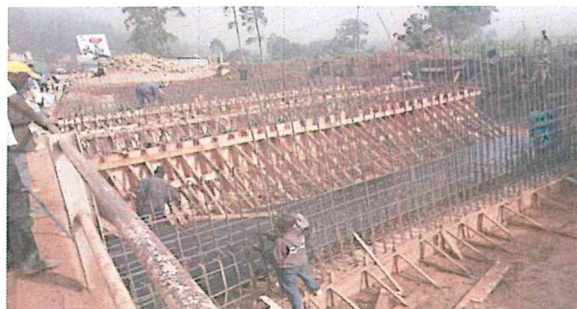
Figure 5: On-going construction of a bridge at Gatuna OSBP.
