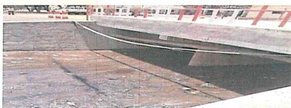
Figure 4: Bridge at Gihengeri connecting Nyagatare and Gichumbi District
