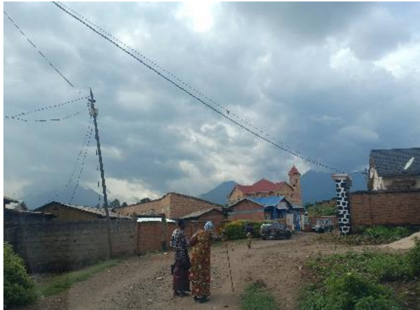
Plate 4-5: Affected structure and electricity distribution mains.
